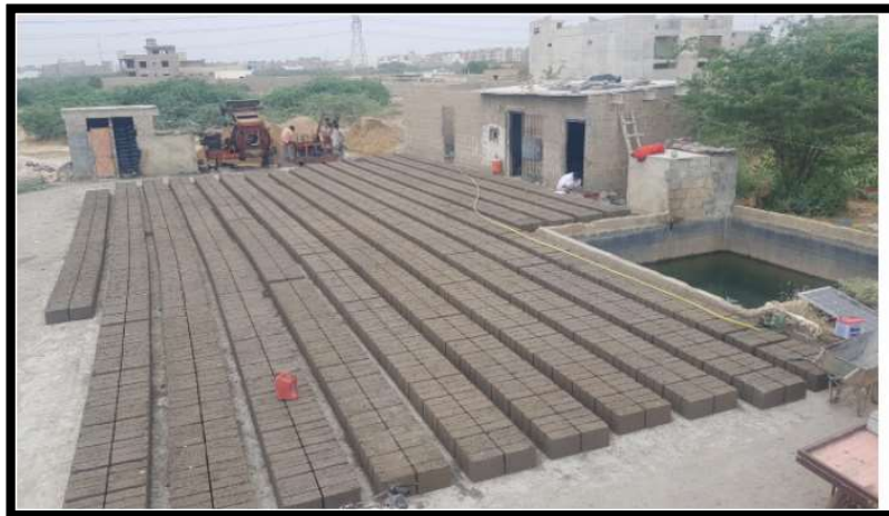
MCC Block Manufacturing Unit,
